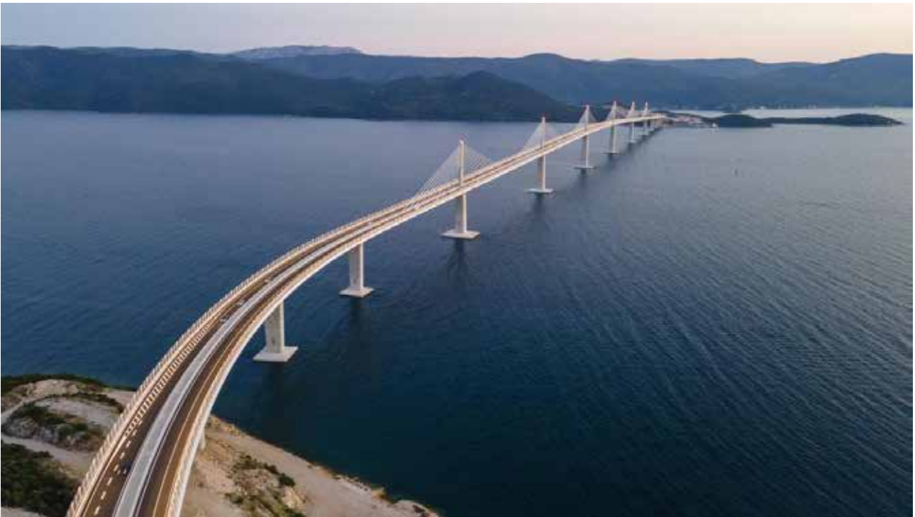
Panoramic view of the Pelješac Bridge.
