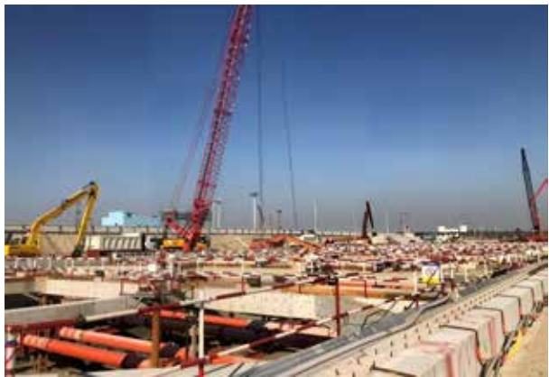
On-site construction photo
