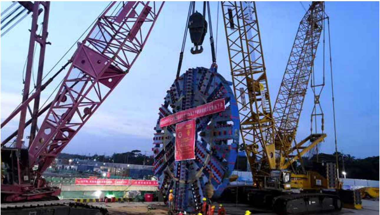
TBM assembling on site
