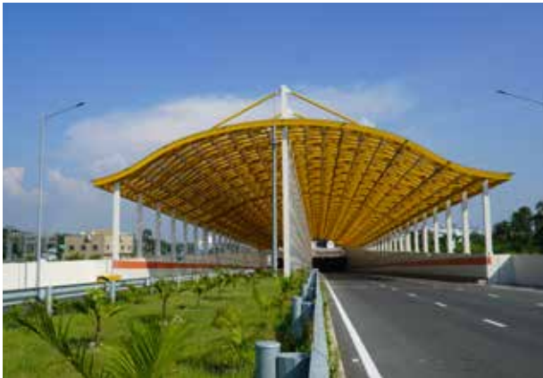
The port of the tunnel
