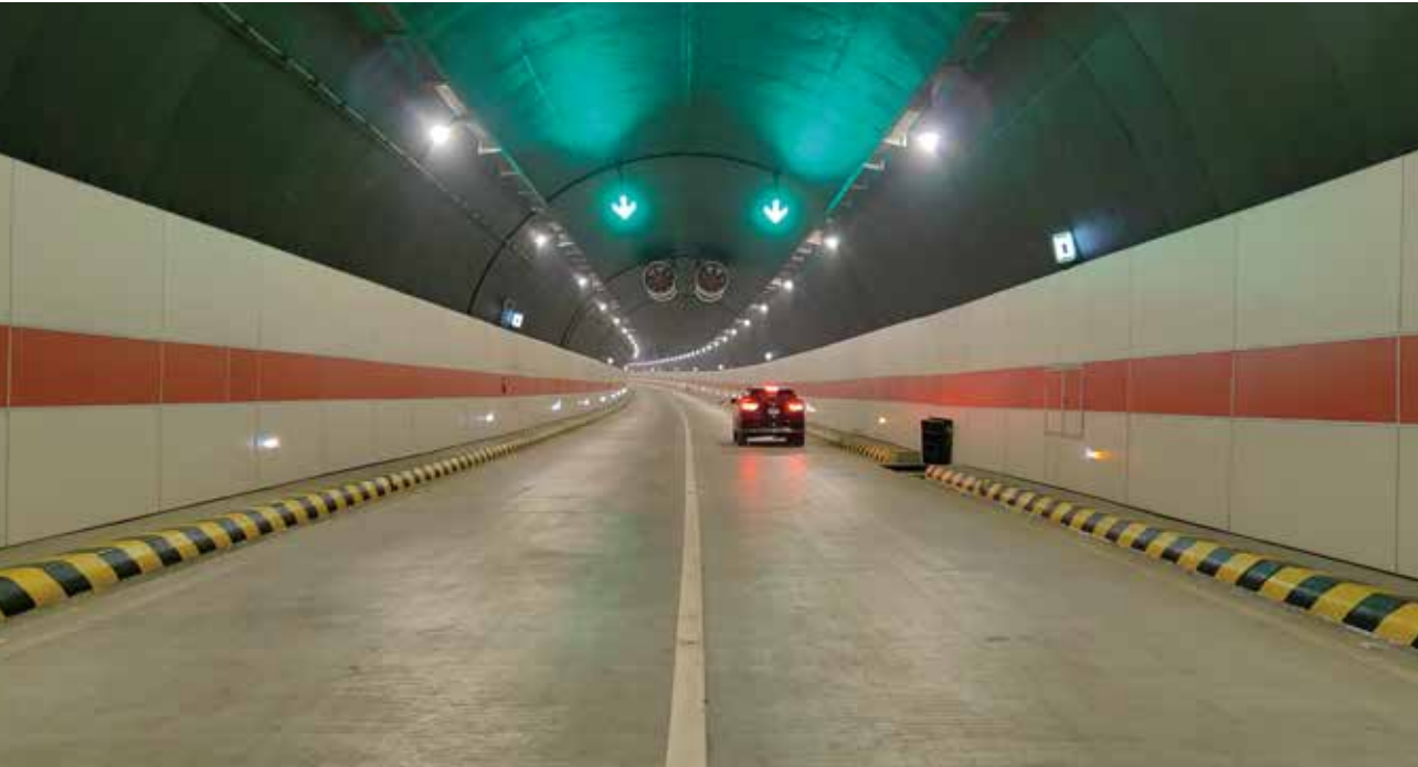
Inside vision of the tunnel
