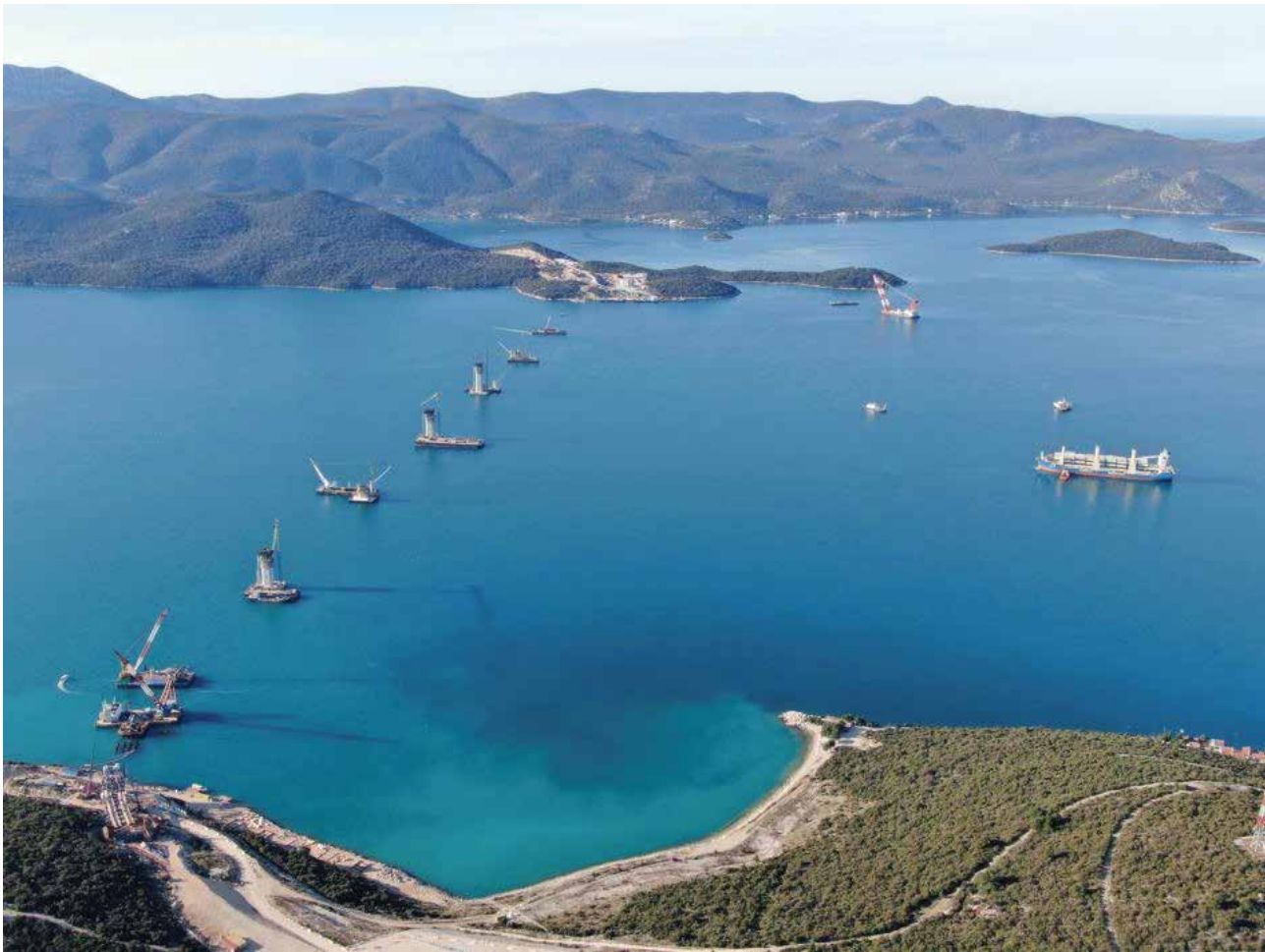
Construction works in the marine environment during the Pelješac Bridge project.
