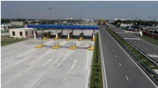
Overload control station on the west bank
