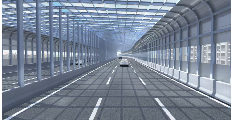
Full-enclosure noise barriers on the section of the Shanghai-Jiading and Jiading-Minhang link lines that passes close to residential areas and schools
