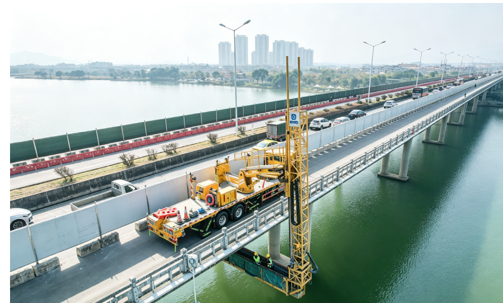
Construction site of the reinforcement and rehabilitation project on the Zhangzhou Bridge along National Highway 324
