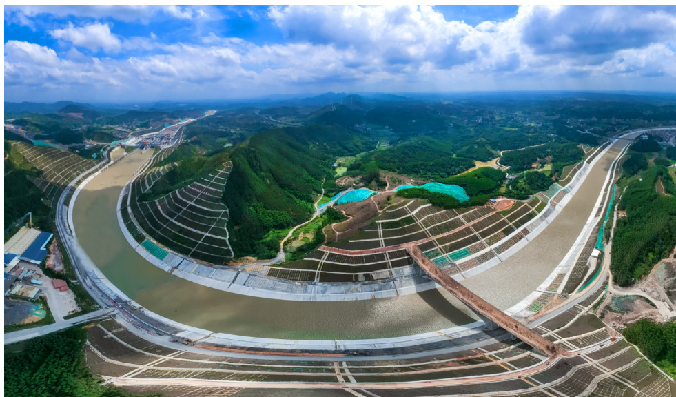
Wildlife crossing bridge on the Pinglu Canal
