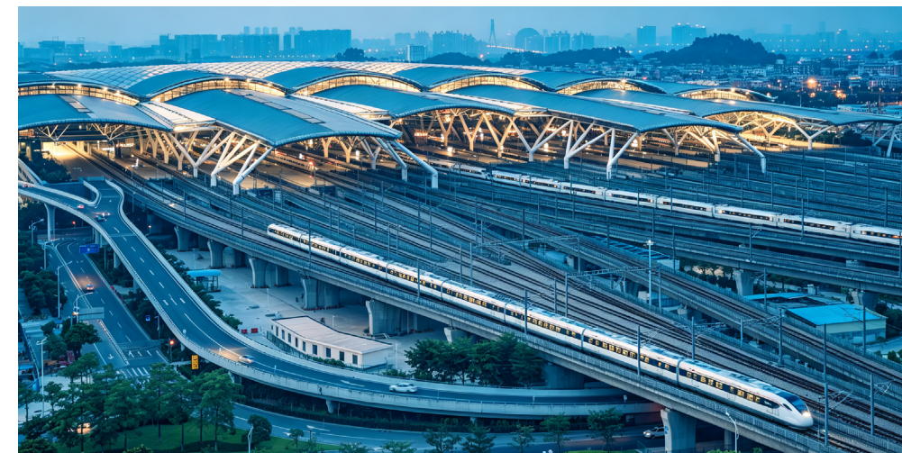
Guangzhou South Railway Station
