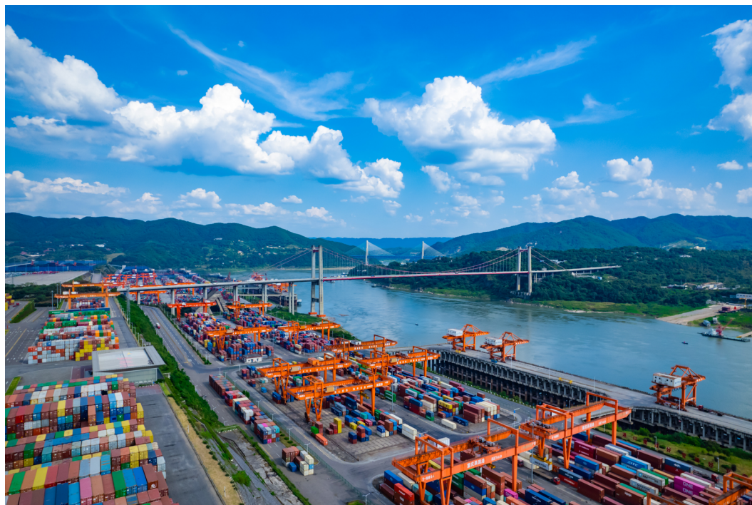
Guoyuan Port in Chongqing, a rail-road-water multimodal transport hub
