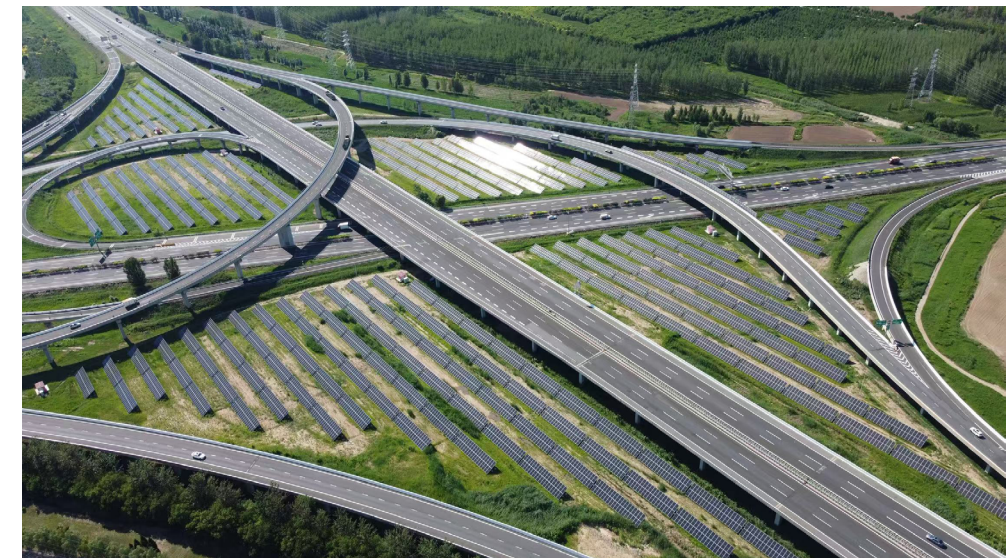
Tianjin-Shijiazhuang Expressway photovoltaic project
