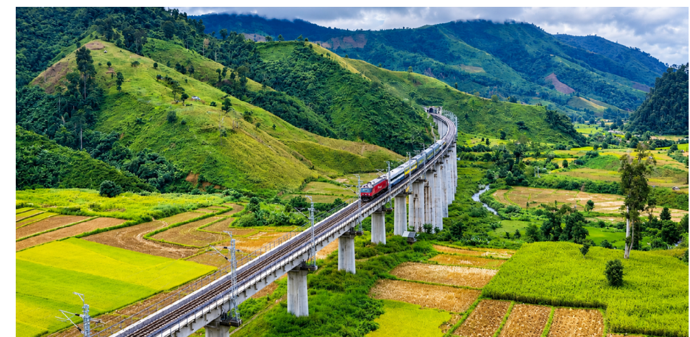
The Nangai River Grand Bridge on the China-Laos Railway
