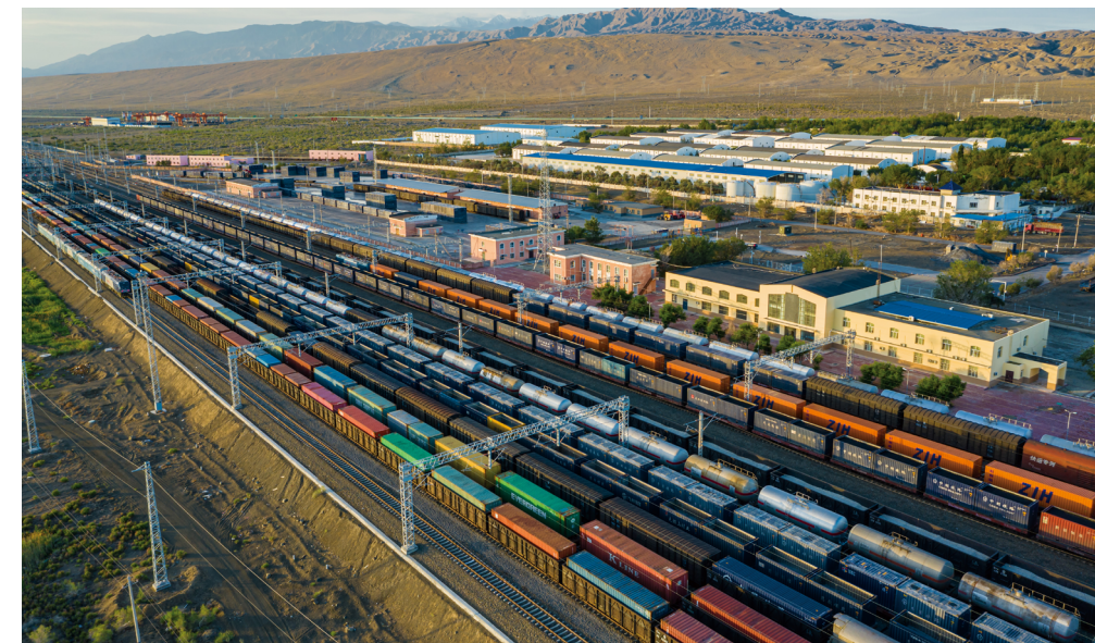
China-Europe Railway Express freight yard
