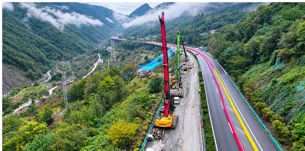
Crews installing rail piles during the emergency repairs
