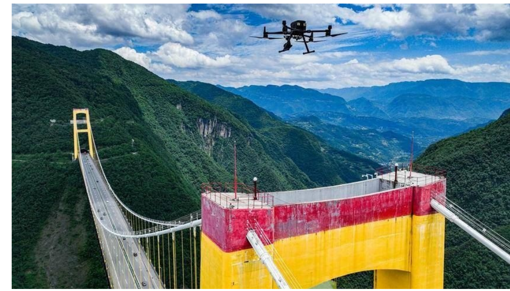
Automated drone inspection of an expressway bridge
